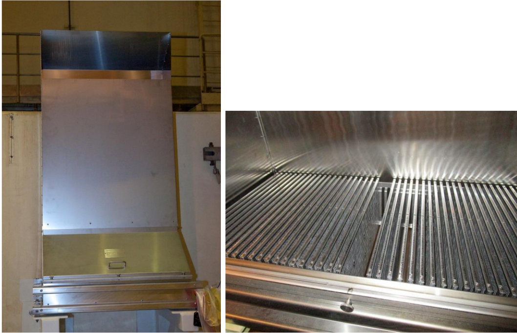
Figure 1: An example of the PAR unit installed in NEK
