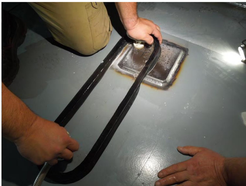
Figure 6: Vacuum box inspection of welded patch
