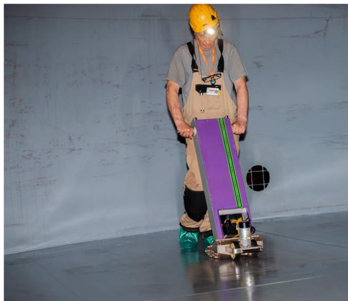
Figure 5: Inspection of bottom plates using MFL detection scanner.
