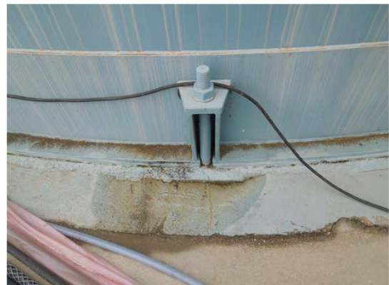
Figure 1: Condensate storage tanks 1 and 2 Figure 2: Possible signs of leakage on tank 1
