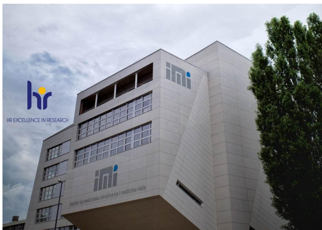
Figure 1: New IMROH building
