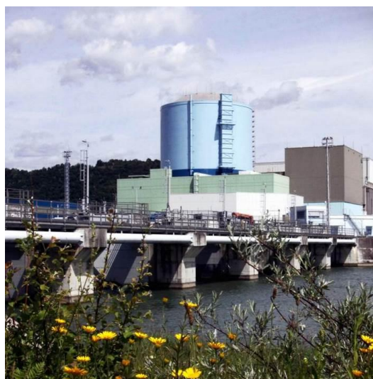
Figure 1: NPP Krško (NEK) with its class MC containment building. (Photo: R. Germovšek)
