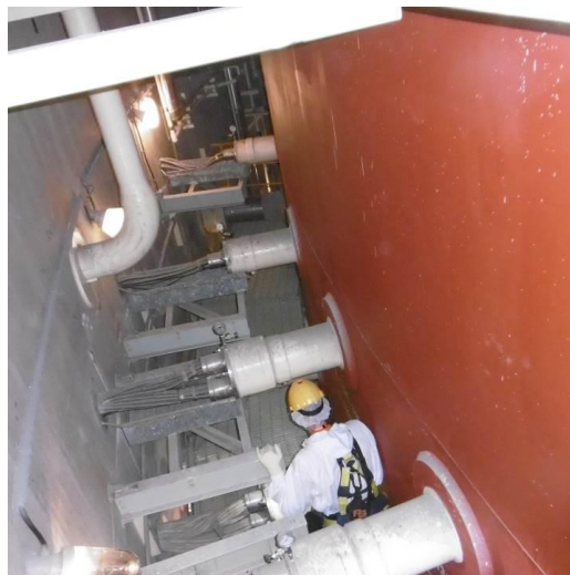
Figure 5: Detail from inspection, electrical penetration area.
