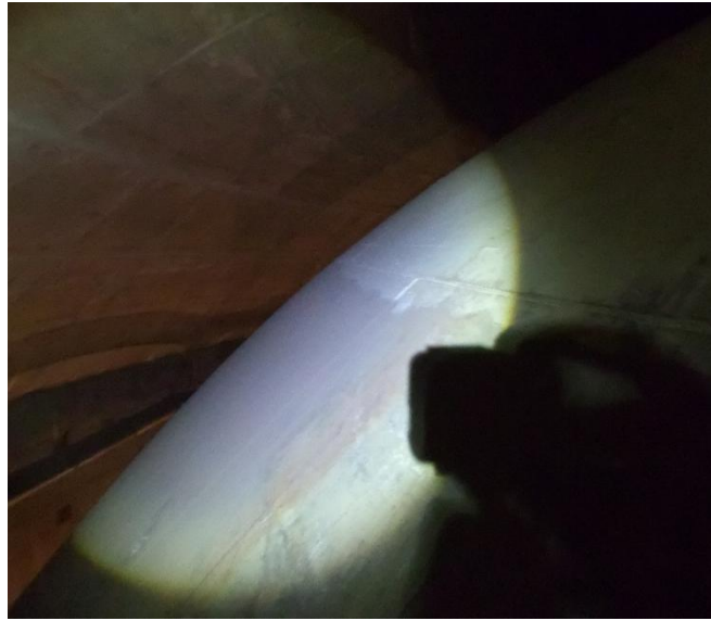
Figure 10: Unpainted part of the containment dome, no development or progression of corrosion due to dry atmosphere.
