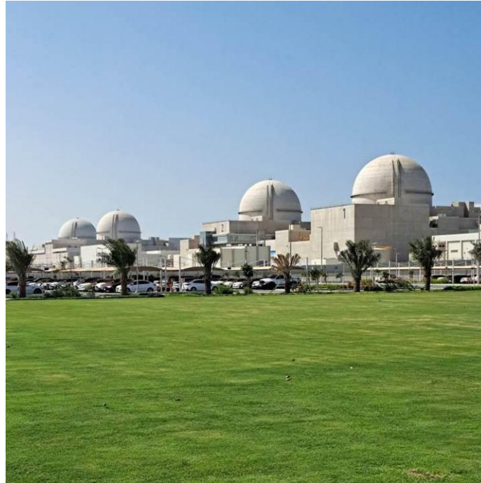
Figure 2: NPP Barakah, 4 units with class CC containment buildings. (Photo: L. Pušnik)
