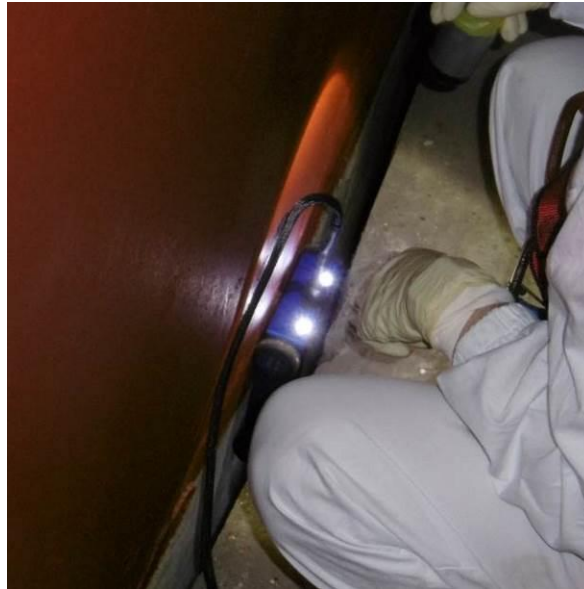
Figure 7: Inspection of gap behind a concrete neutron shield wall with remote-controlled crawler in 2022.
