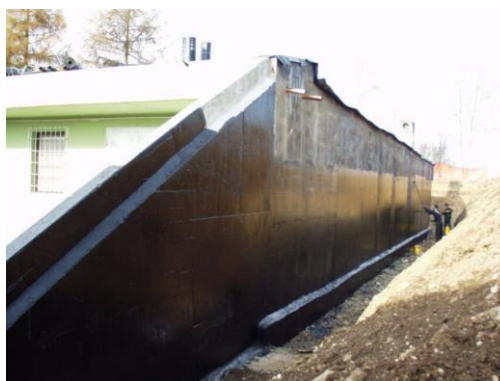
Figure 2: Renovation of the facility's hydro-isolation in 2001
