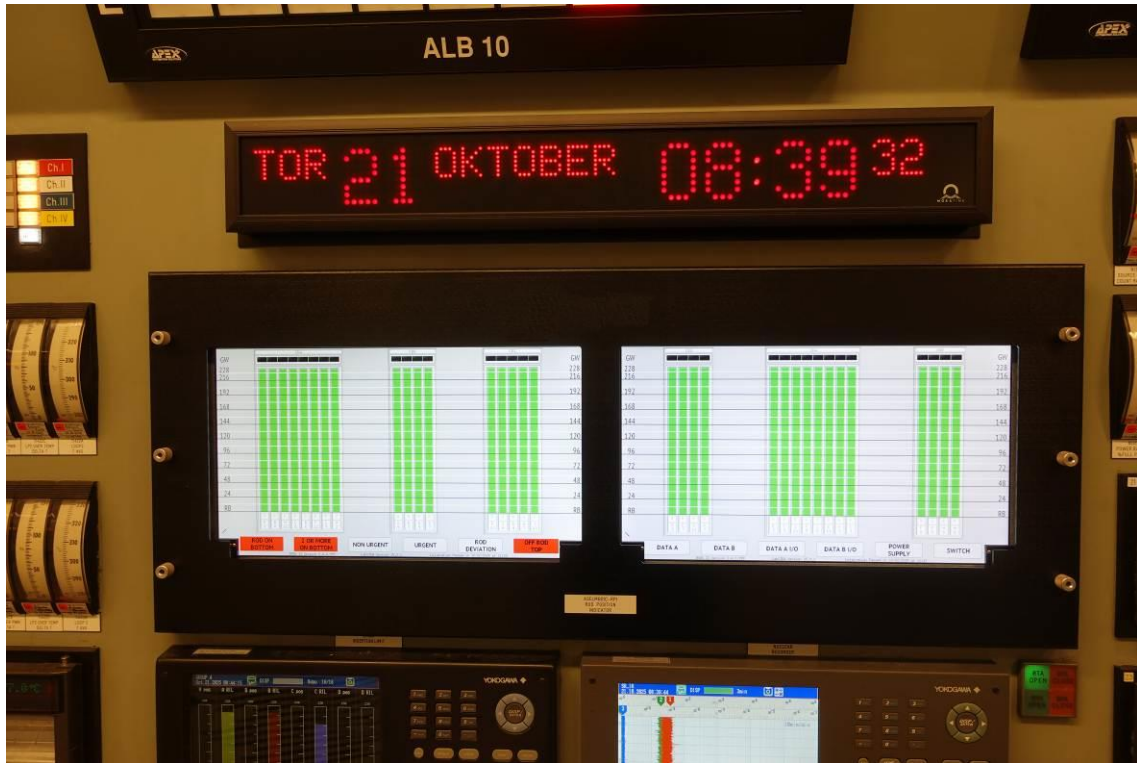
Figure 3: New DRPI displays with NEK configuration
