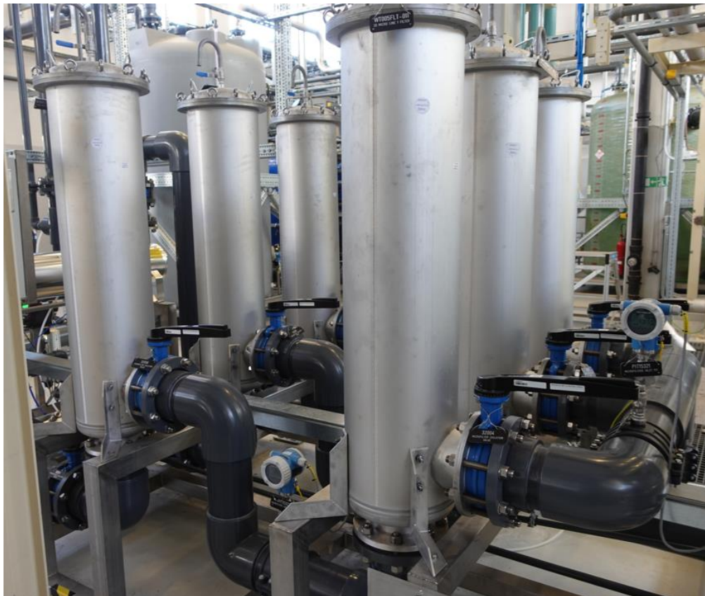
Figure 2: Microfiltration Skid
