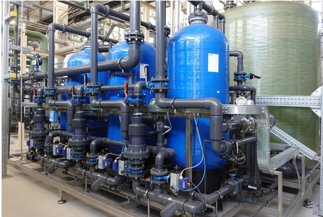
Figure 8: Polishing Mixed Beds
