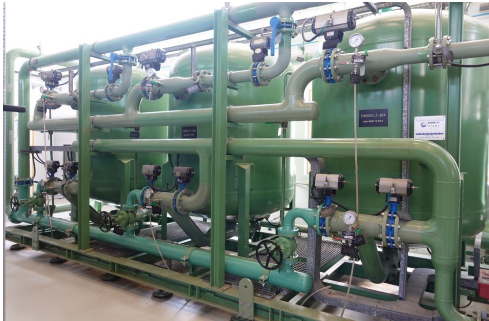
Figure 1: Sand Filters
