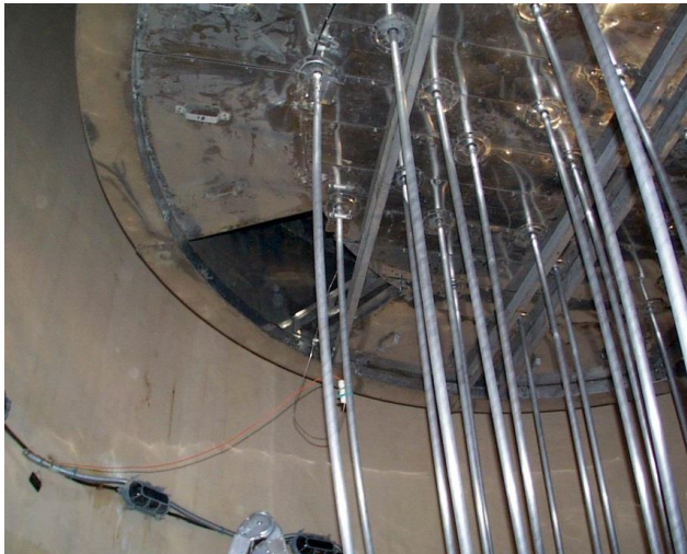
Figure 8: NPP Krško RPV insulation details (2) – incore syst. penetrations
