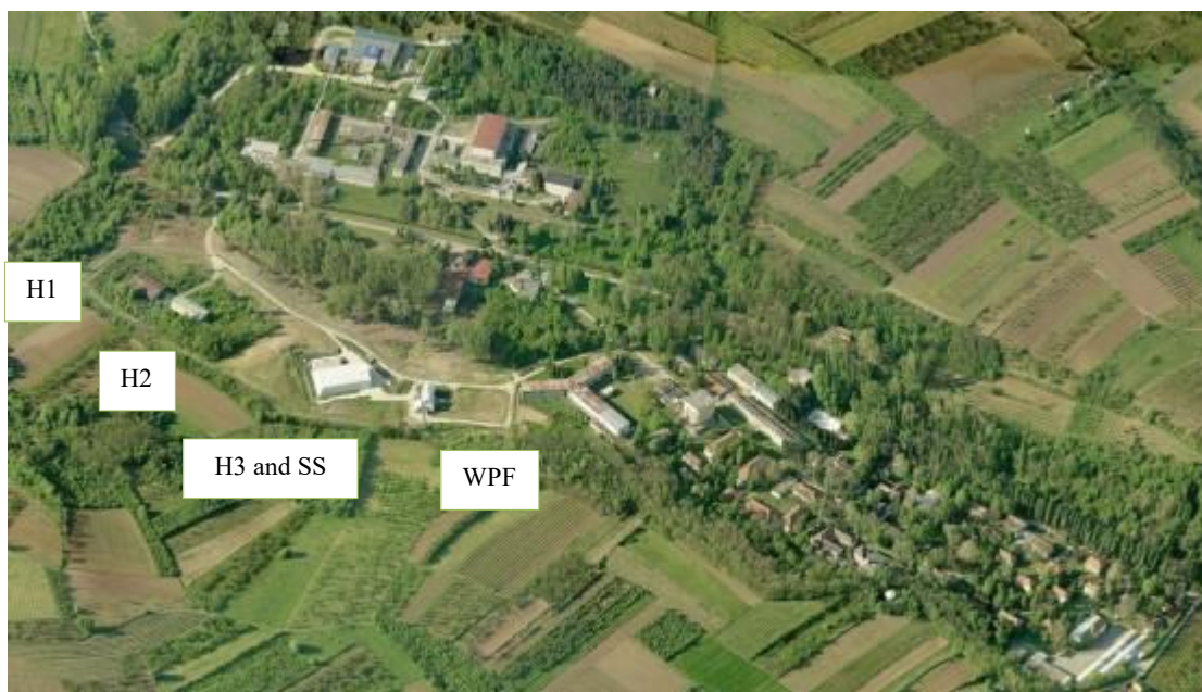
Figure 1: Disposition of the RW facilities, old hangars H1 and H2, new hangar H3 and SS, and WPF
