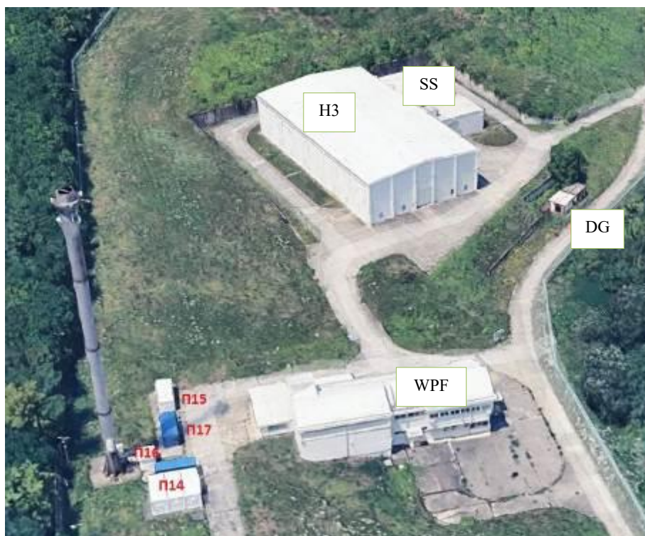
Figure 11: Operational radioactive waste management facilities H3, SS, DG and WPF
